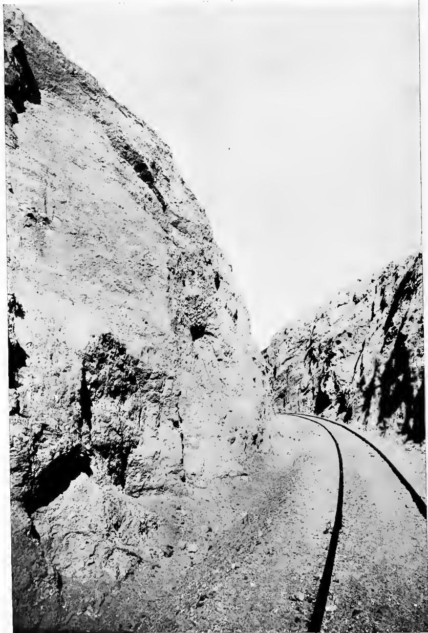
ONE OF THE DEEP CUTS ON THE ARICA-LA PAZ LINE.
